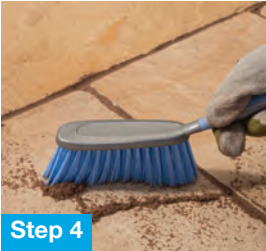
Step 4 Refill, if necessary, using a small soft hand brush.
