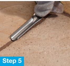
Step 5 Compact the surface to give it a clean flat finish.
