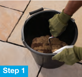
Step 1 Open both packs, measure 50/50 ratio of each & mix until uniform in colour.
