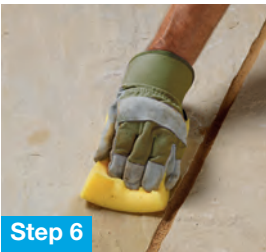
Step 6 Brush off any excess & wipe off any remaining residue with a damp sponge.
